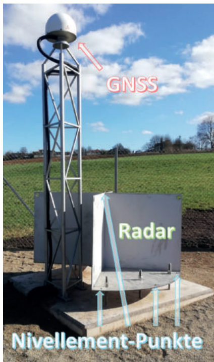
Fig. 7: Radar control point in Saarland (Eft-Hellendorf station, Perl).
