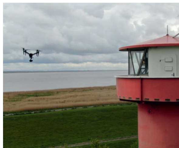
Fig. 5: UAS deployment in WSV. Source: WSA Elbe-North Sea
