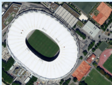
Fig. 34: Orthophoto as HVD with a ground resolution of 20 cm, Mercedes-Benz Arena. Geospatial reference data © LGL, www.lgl-bw.de
